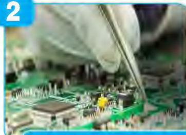
Solar Charging Controller Inspection
