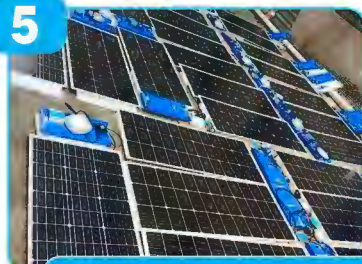
Semi-finished Parts Testing Together
